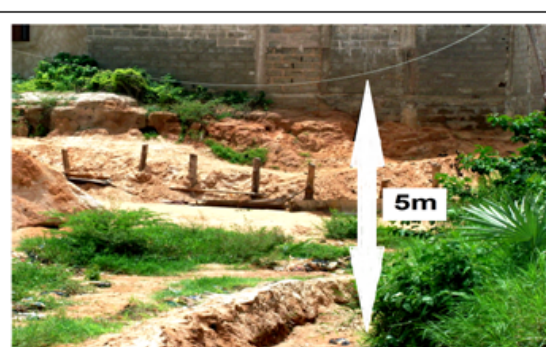
b- Erosion has transformed the road into a duct of more than 5 m deep leading to the collapse of houses.
