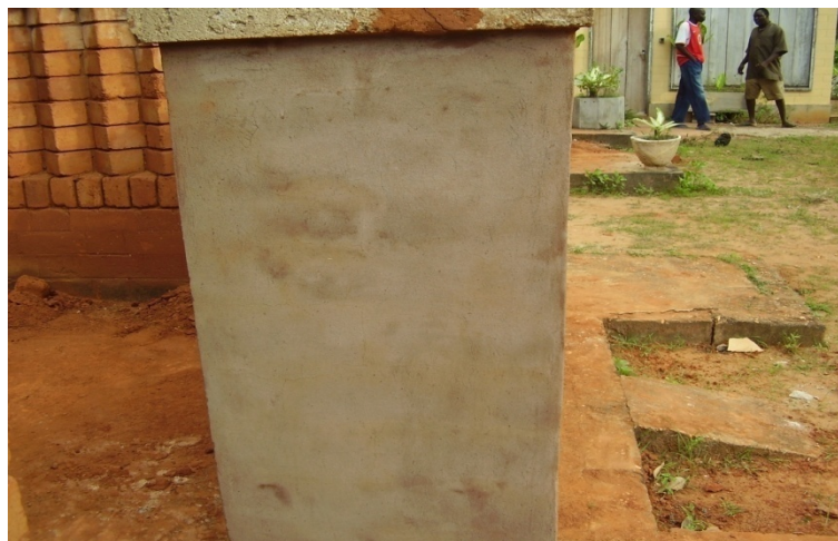
Fig. 3 Micro clay coating, sand, cement and locust bean fruit husk's extract.
